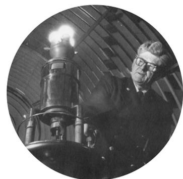
When the optic went into Mew Lighthouse, the fuel to produce the light was changed from gas to paraffin. The new paraffin lamps had three ceramic mantles which encased the flame and produced a bright white light equivalent to 1,210,000 candles.
