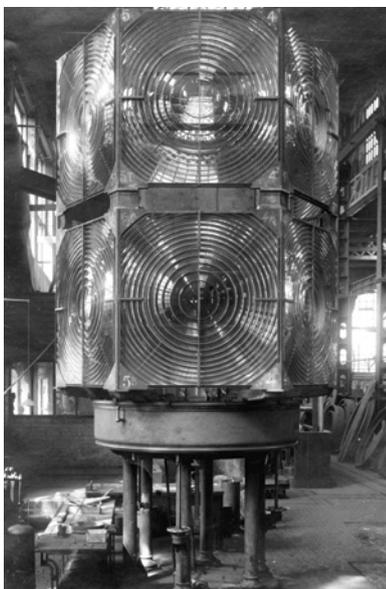
In the 1920s the Tory Island optic was taken out of its tower and sent to the Chance Brothers in Birmingham. It was changed to a biform (two tier) optic with four lenses and two blank panels per tier in a hexagon formation, with a new pedestal and sent back to Tory lighthouse.
