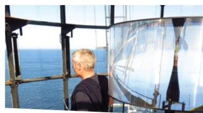
On 21 November 2014 the light was changed to a light emitting diode (LED) powered by renewable energy from solar panels. The light was equivalent to 63,400 candles. The lighthouse also had a radio beacon and an Automatic Identification System (AIS) and therefore did not rely on strong light.
