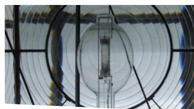
Generators were brought to Mew Island (1972 on Tory Island) to produce electricity. The paraffin lamps were changed to 3.5 kW electric lamps which produced light equivalent to 5 million candles and could be seen, on a clear night, 30 nautical mile away (a nautical miles is equivalent to 1,852 metres). The clockwork mechanism rotating the lenses was replaced with an electric motor.
