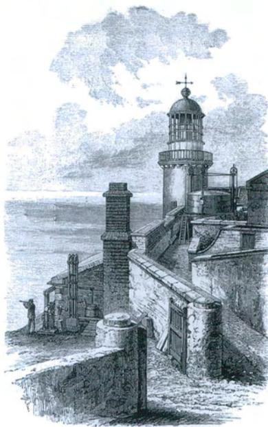
Wicklow Head Lighthouse, gas holding tank at the right of the lighthouse. Drawing from the author's collection.
