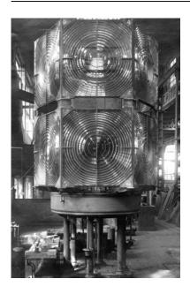
In the 1920s the Tory Island optic was taken out of its tower and sent to the Chance Brothers in Birmingham. It was changed to a biform (two tier) optic with four lenses and two blank panels per tier in a hexagon formation, with a new pedestal and sent back to Tory lighthouse.
